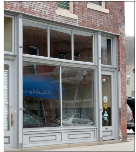
Many downtown building retain a high degree of integrity as historic resources.
