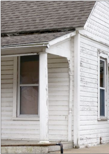
Priority: Target programs to encourage rehabilitation of residential buildings.
