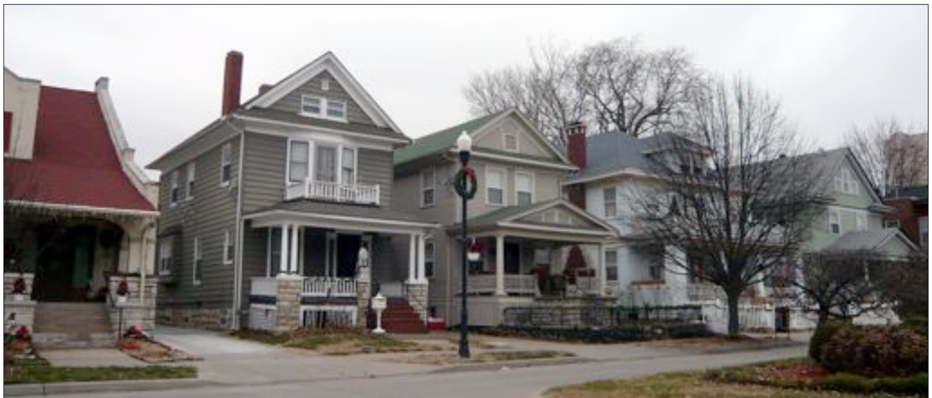
The potential Oak Street Historic District
