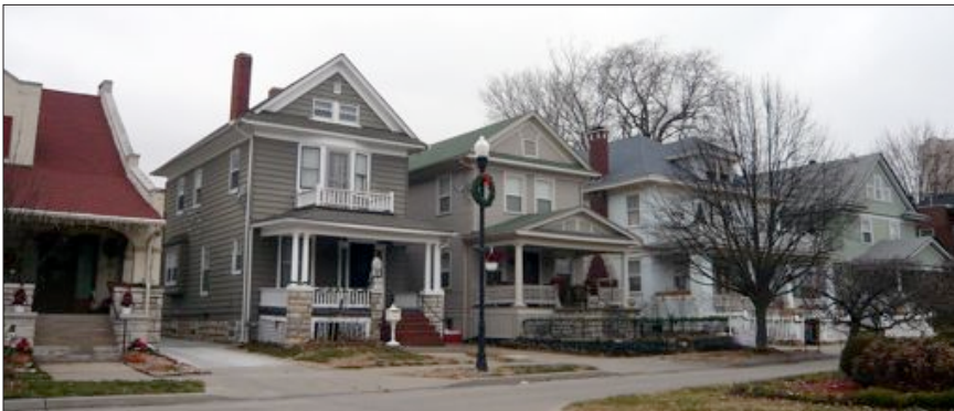
The potential Oak Street Historic District
