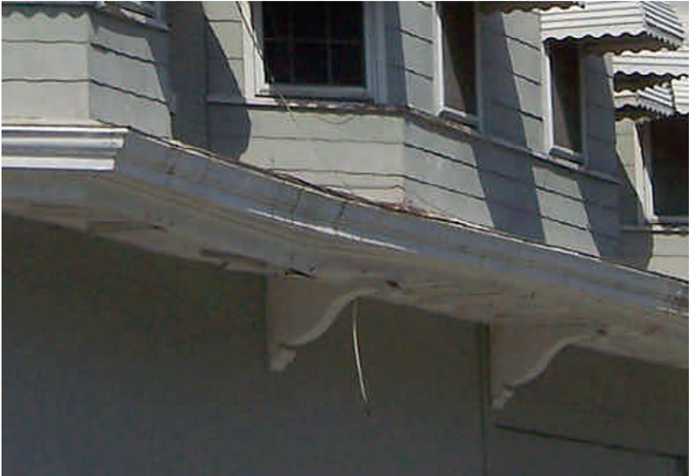
Original soffit at 208 Spring Street
